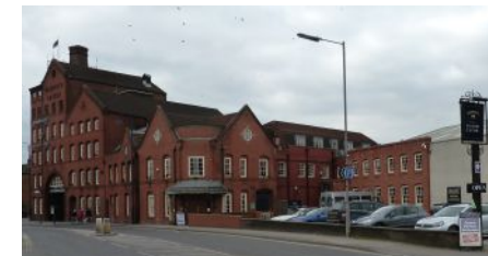
Wadworth Brewery Visitor Centre
